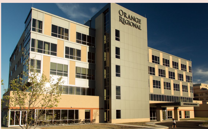
Orange Regional Medical Center's 153,000-square-foot, five-story outpatient building opened in September.
